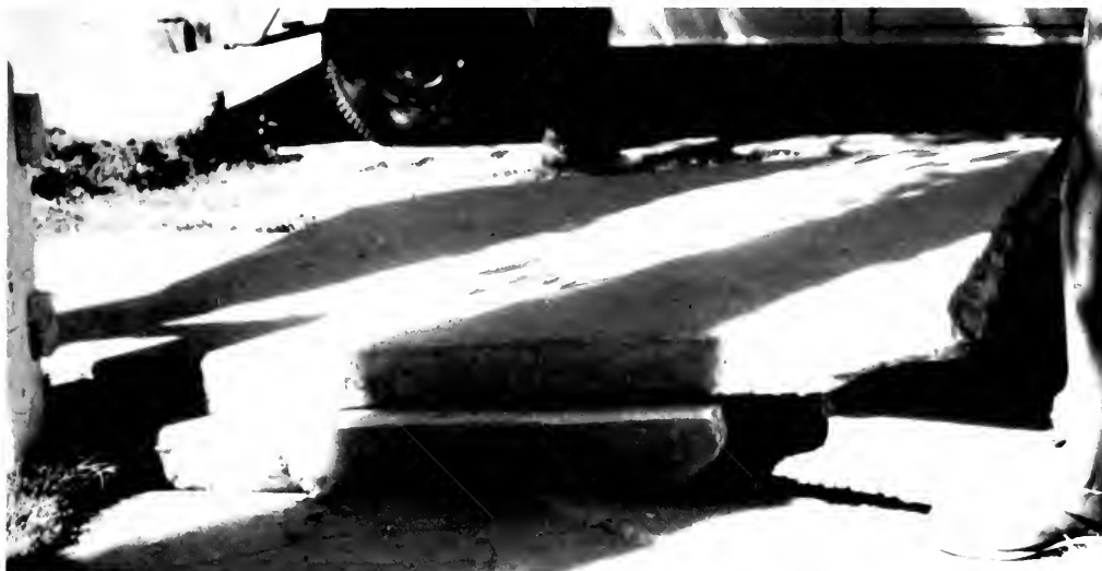
Photo 5. Ejected slab in sidewalk at corner of Orange Grove and Phillippi in Sylmar fault zone. Fault thrusting caused by shortening of continuous sidewalk along block by about 2 m.
